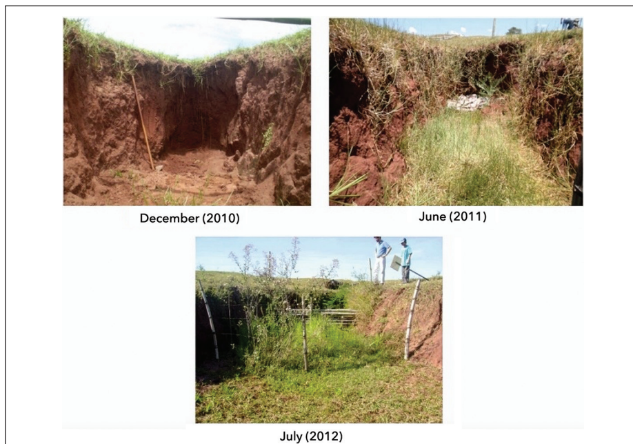
Figura7. Temporal evolution of the erosive process recovery with the combined use of mechanical systems (dam with bamboo) and edaphic systems (planting of native seedlings)
