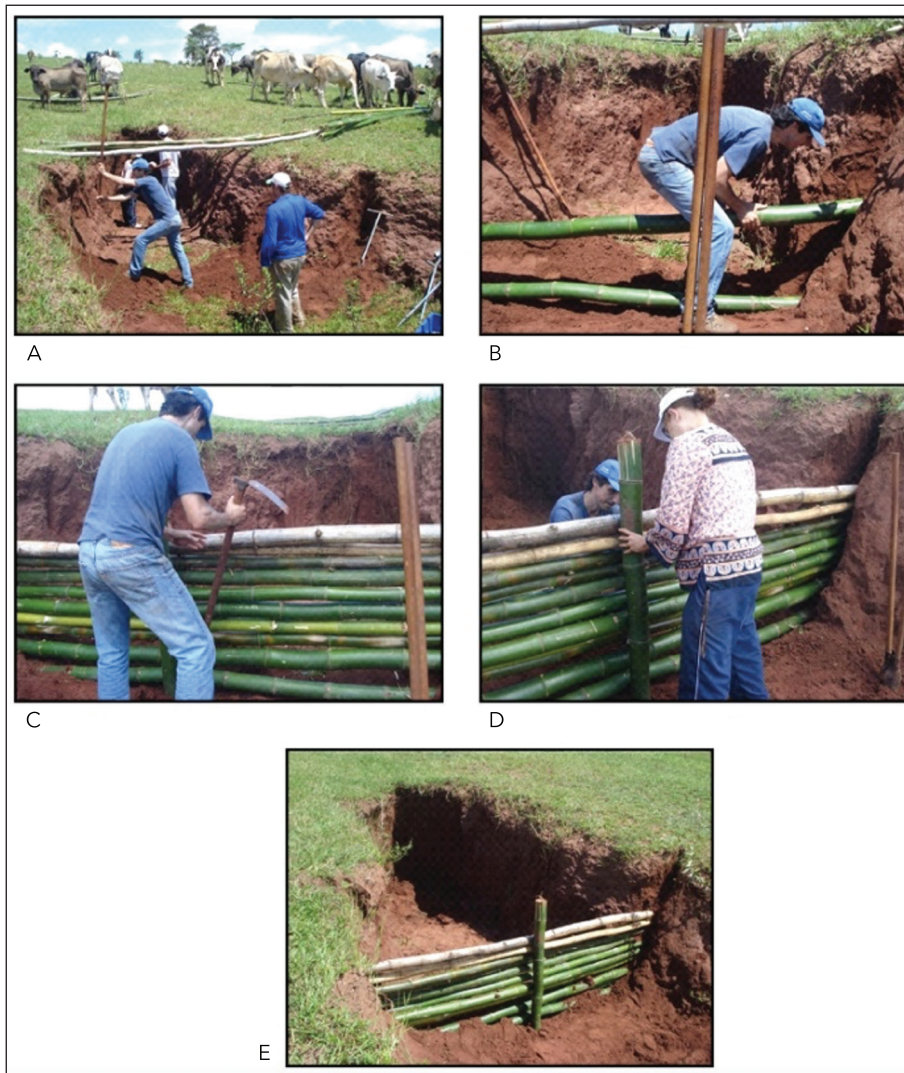
Figura 4. Barrier assembly sequence using bamboo inside the rill erosion (June 2011)
