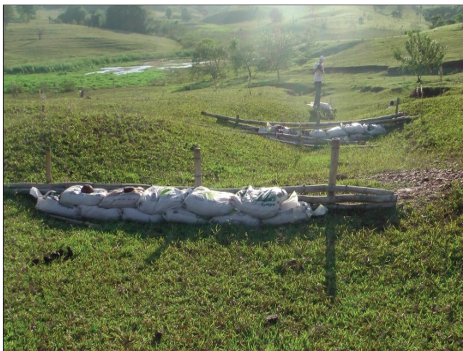
Figura 3. Barriers made with raffia bags (sand and pebbles) supported by bamboo, upstream of the erosion (June 2011)
